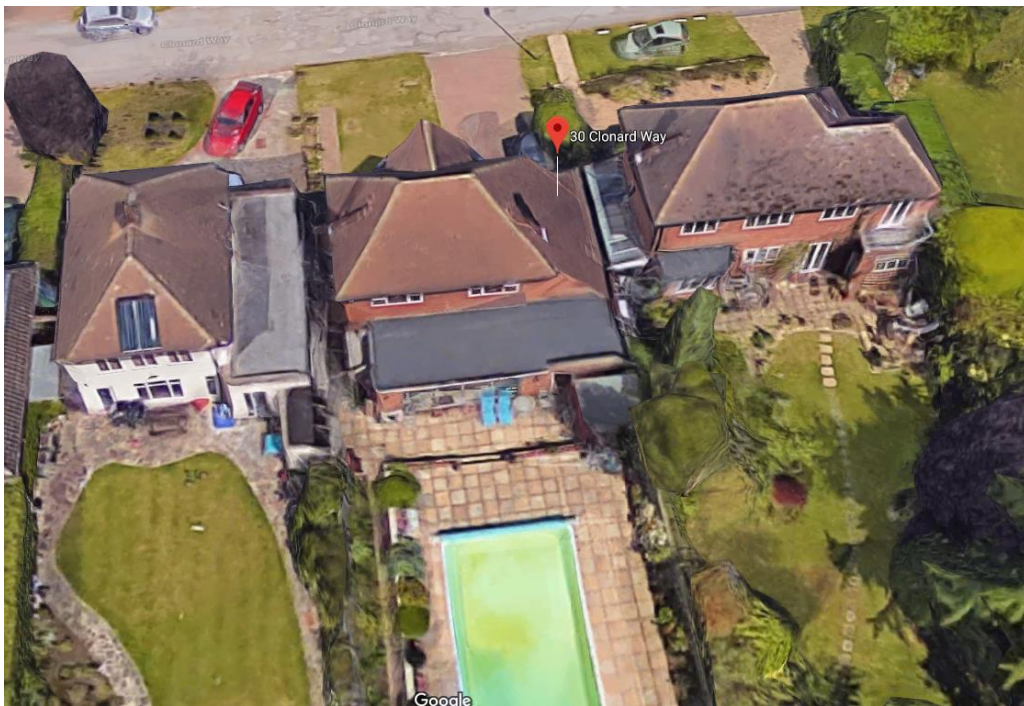
Google image- rear elevations
